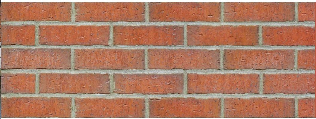
Brick tower HF03
